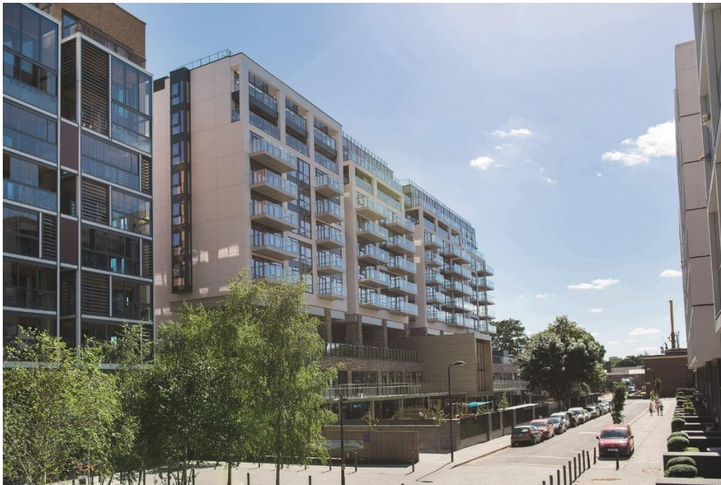
Telford Homes' Holy Trinity Primary School / Vibe, London E8
